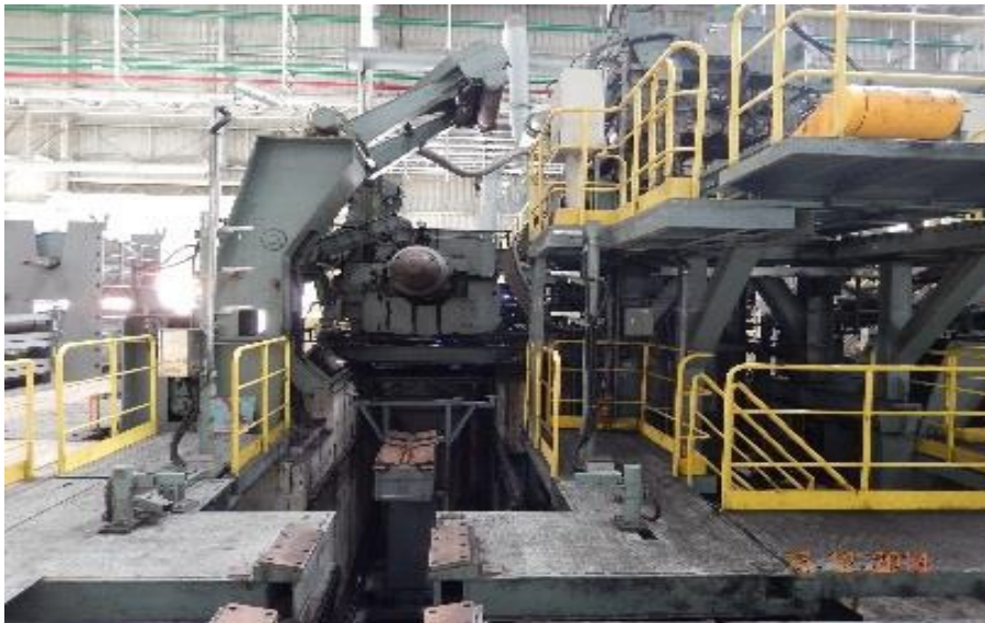
Picture 1: Two Pay-Off Reel In The Entry Section
